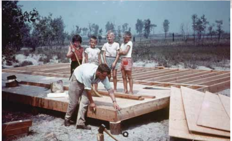
David Hussell and supervisors working on the Tip cabin.
